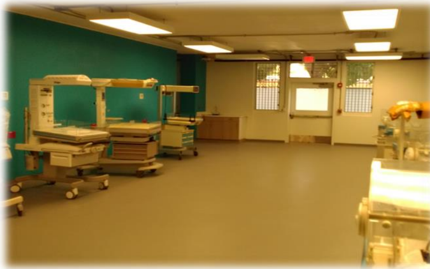
Figure 6. Hospital Justinien, Pediatrics Section. New Building with Equipment Not Installed
